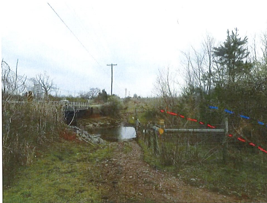
Photo 2.1 Facing east towards bridge showing approximate edge of take (red-line) and temporary easement disturbance (blue-line).
